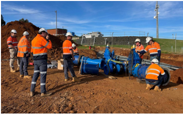
Burnie Trunk Main Renewal
