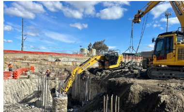
Launceston Sewer Treatment Storage Tank Earthworks and Pile Cropping
