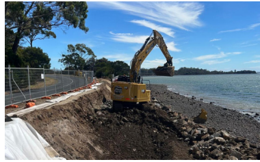
Beauty Point Foreshore Seawall Restoration
